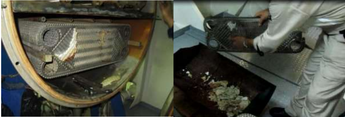
Figure 9. Some plates had limescale on them, but it was easily removed by hand
