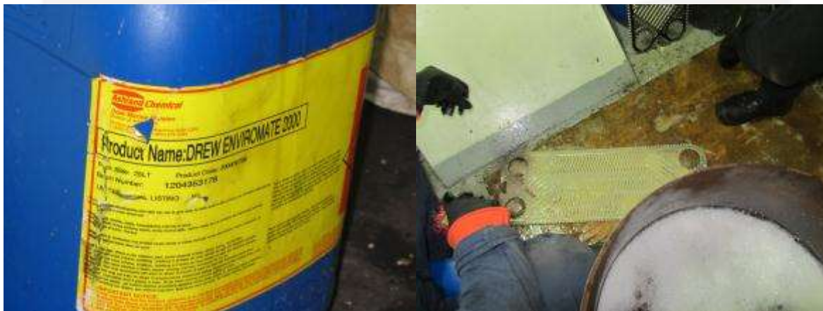
Figure 4. Left: Drew Enviromate 2000 – multipurpose cleaning. Right: Plate is brushed to remove dirt.
