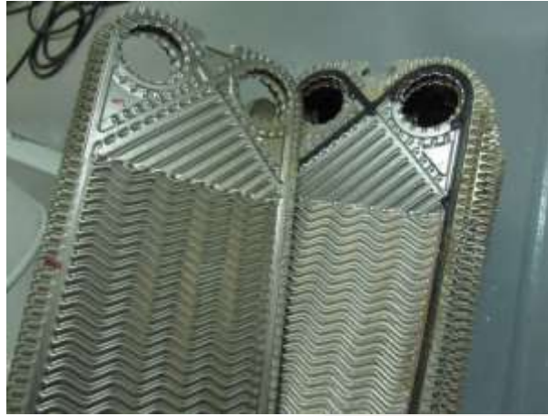
Figure 11. June 2013 – after installation, of the HydroPath MARINE unit the plates are clean.
