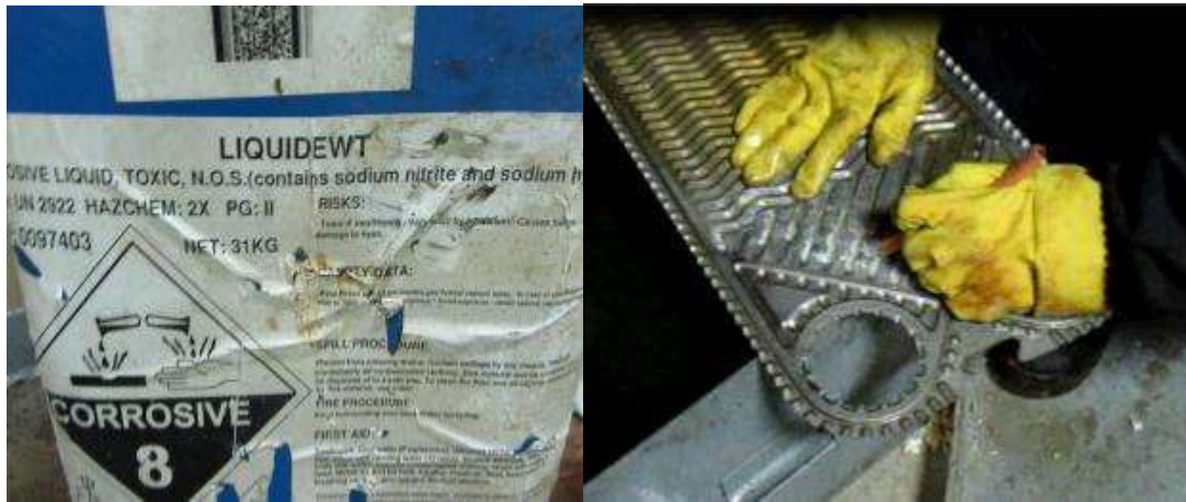
Figure 5. Left: Chemical used to soften limescale. Right: Carving out limescale
