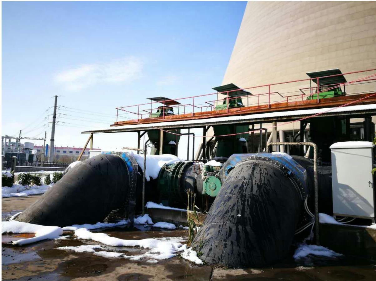
This application was on an inland power plant in China, which used water from the Yuen for the cooling system of 2x 600MW. The inlet pipe to each of the two condensers was 1800mm outer-diameter.
